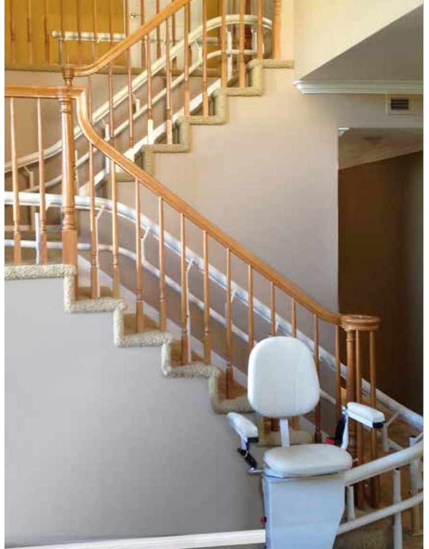
Beige rail with wide 180° turn the landing of the banister side of stairs
