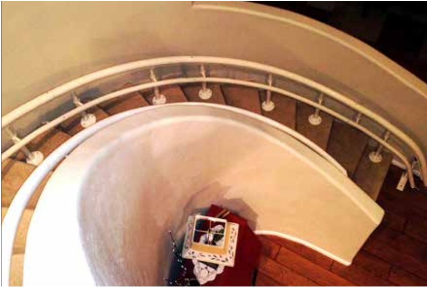
Beige rail with long sweeping turn on the wall side of the stairs
